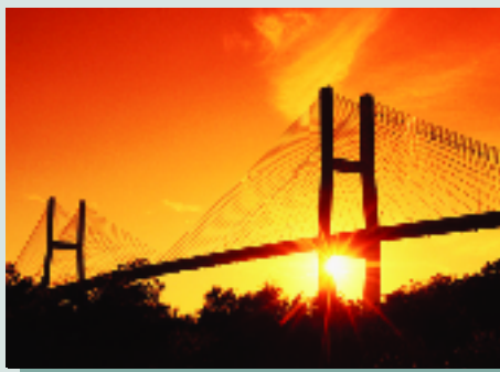
Bridges and Flyovers
