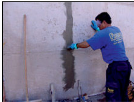
hairline cracks were simply treated with a coat of Penetron slurry
