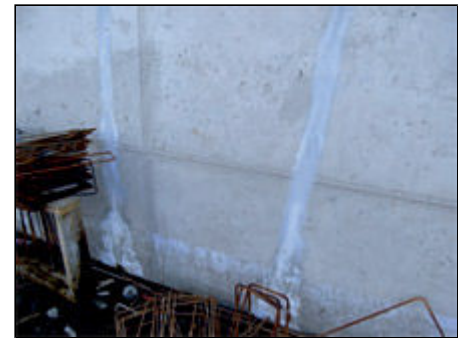
crystal growth after 4 days, no water leakage
