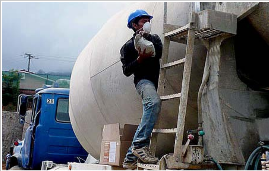
Addition of Penetron Admix soluble bags
