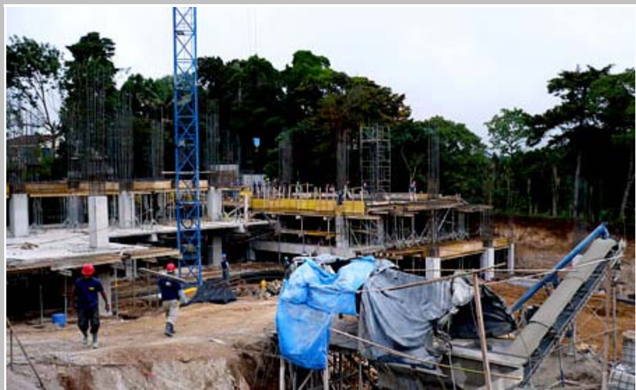
Verdino Project Site
