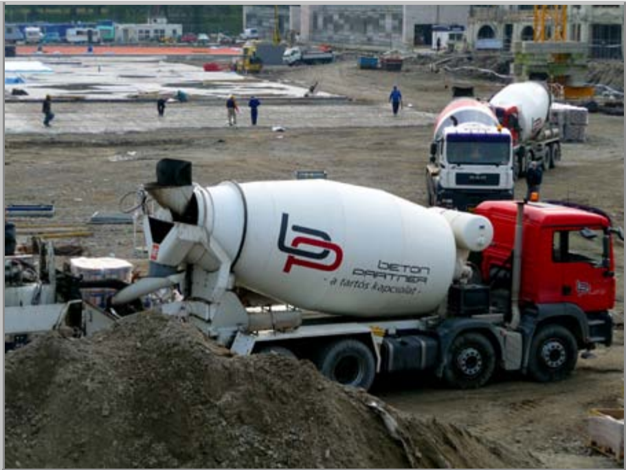
Concreting with Penetron Admix on site
