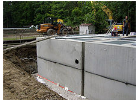
Site works at Lakeshore
