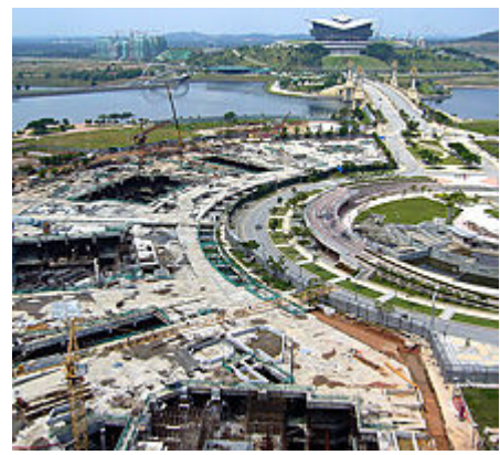
Basement works in Putrajaya, Precinct 4
