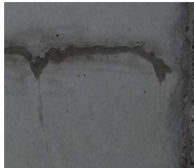
Day 1 Leaks appear as the tank is filled
