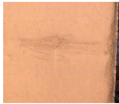
Day 7-All cracks have been filled and leaks completely stopped
