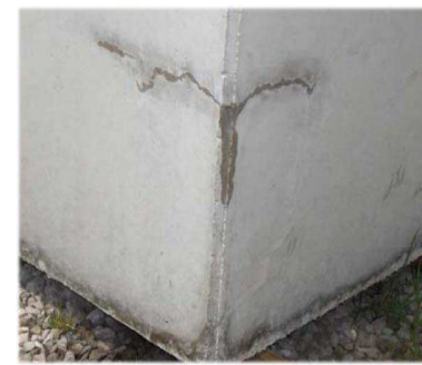
Day 3-Crystals begin to grow filling the cracks
